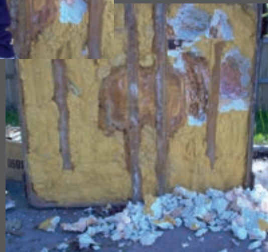
Servicing a foam filled hot tub.
